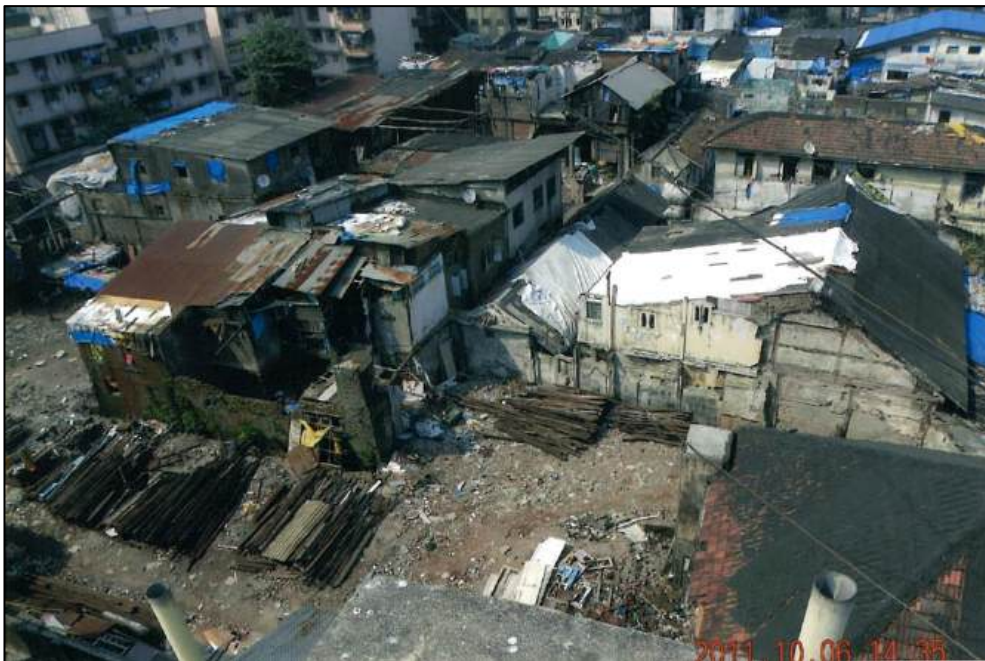
Photo 06/10/2011 before work started at site.
